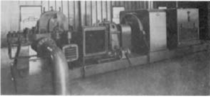
FIGURE 5 Horizontal centrifugal pump driven by a 1000-hp (746-kW), 1780-rpm induction motor through a stepup gear and an eddy-current coupling (Electric Machinery)
