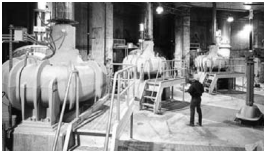
FIGURE 5 Vertical sewage pumping units at the South System Pump Station, Deer Island in Boston, MA containing (8) 36 in (915 mm), 46,300 gpm (10,510 m 3 /h) pumps driven by 1250 hp (932 kW) variable speed motors (Flowserve Corporation)
