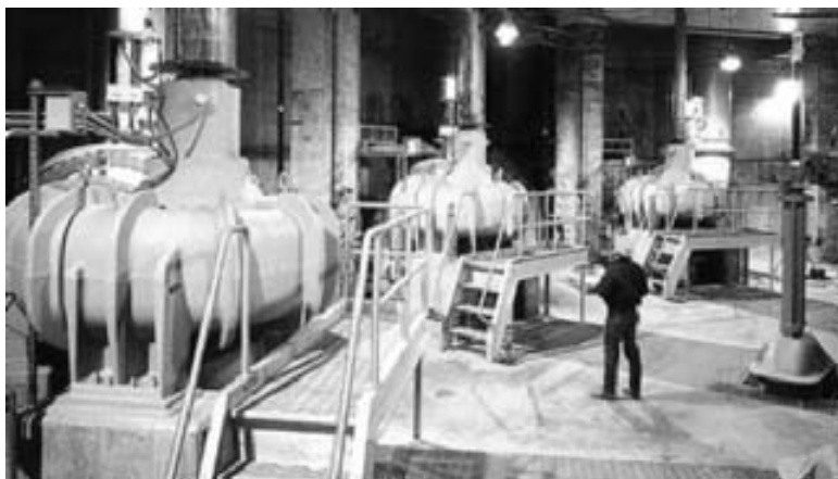
FIGURE 105 Vertical bottom-suction volute pumps installed in a sewage pumping station (Flowserve Corporation)
